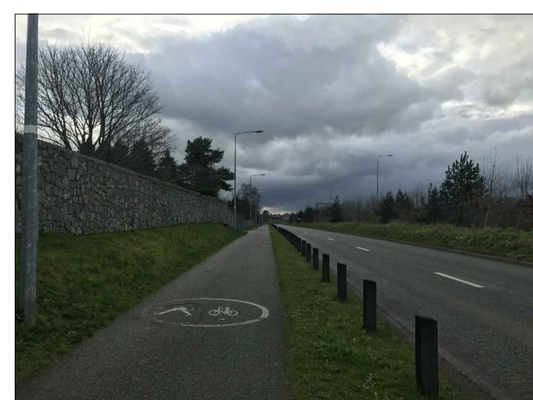
Example of Verge and Wooden Bollards
