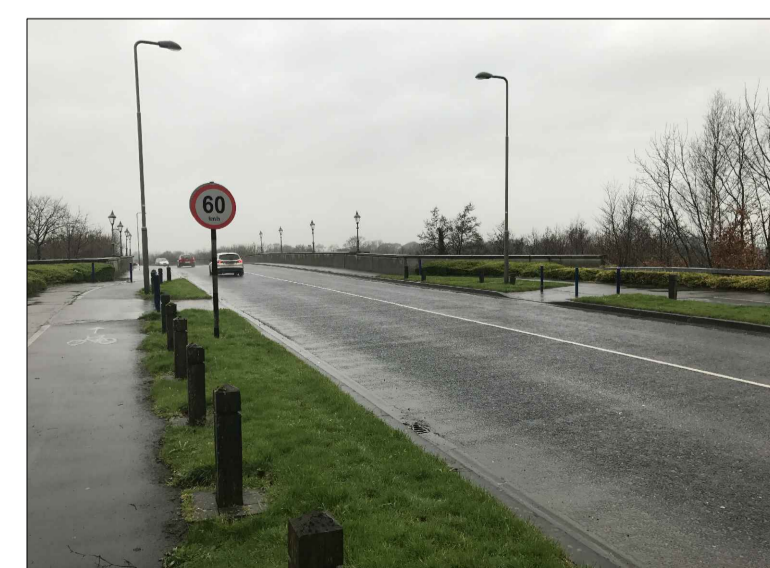
Example of Uncontrolled Crossing at Naas
